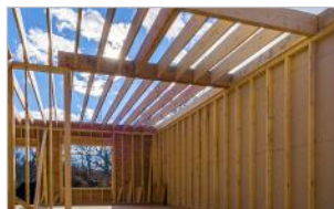
Assemblage ossature bois Wood construction
